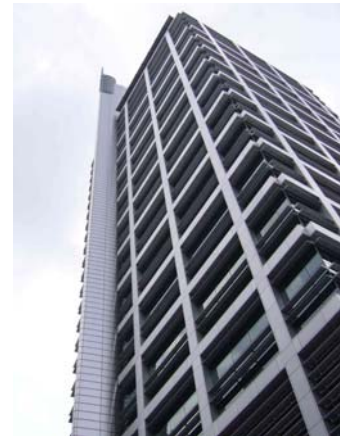
30 Church Street, Singapore SCM is used for vertical fin panels.
